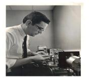
Figure 2 Stickley inserting ruby rod with silvered flat ends into laser head
